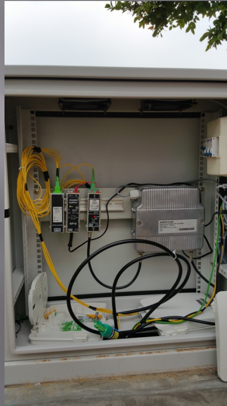
Fracarro Fiber Receivers and Signal amplifiers installed through out Racing circuit
