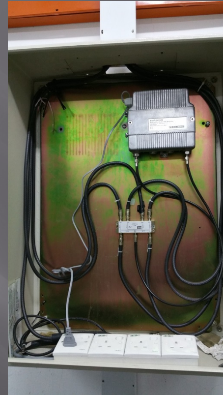
Fracarro Fiber Receivers and Signal amplifiers installed through out Racing circuit
