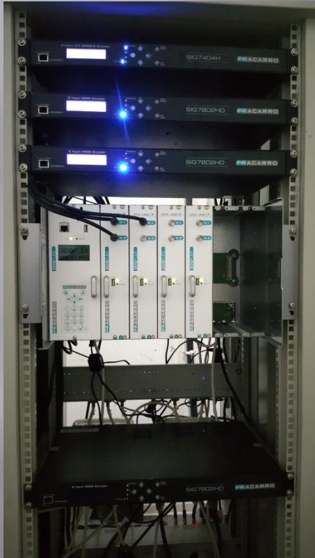
Fracarro 3DGFlex DVB-T headend with Various RCA & HDMI Input Encoders
